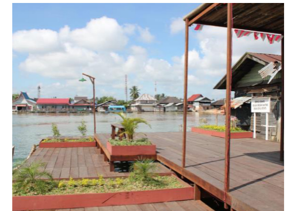
Design and implementation of the public space intervention.
